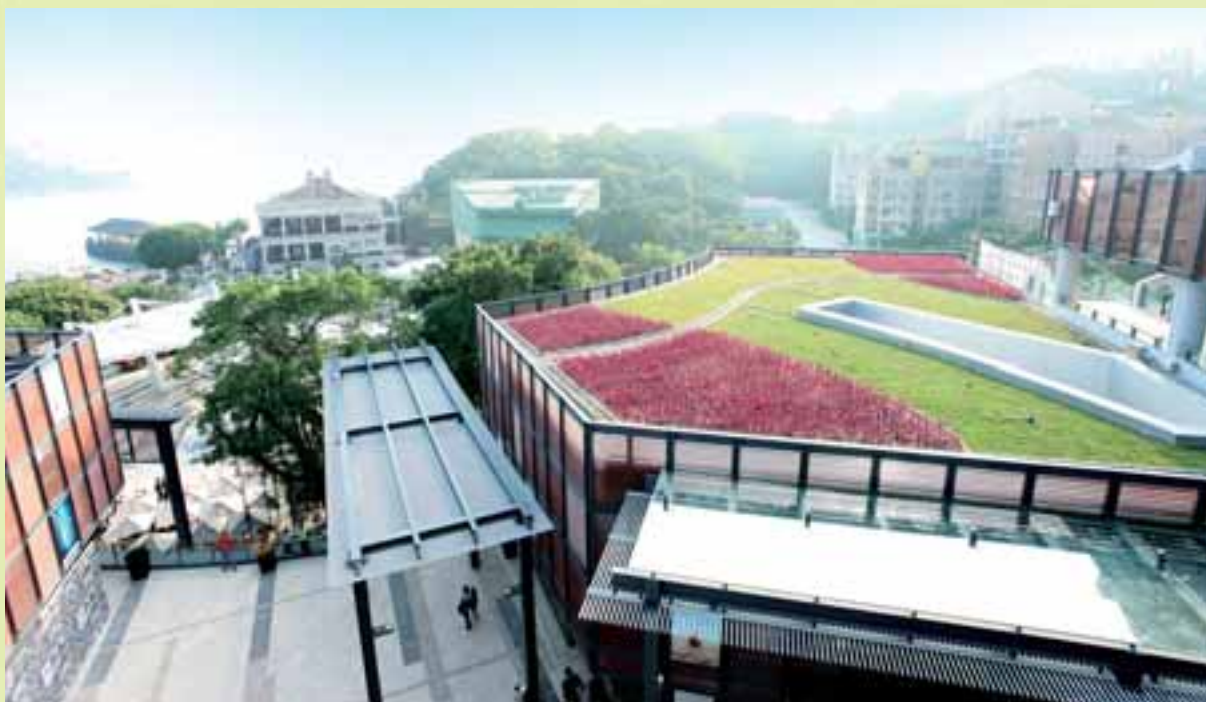
Stanley Plaza's green roof helps reduce heat and electricity consumption
