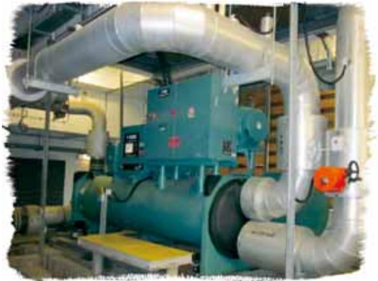
*Energy-efficient water-cooled chiller is progressively introduced at The Link's portfolio*
