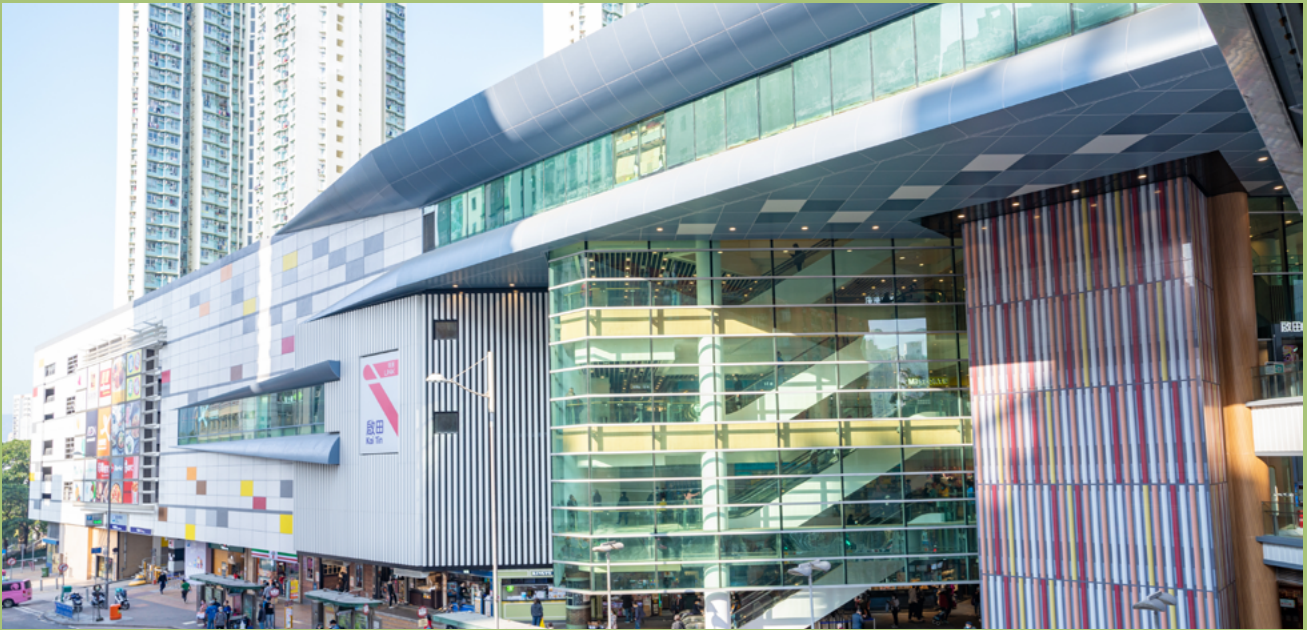
Kai Tin Shopping Centre. (Link Asset Management Limited)
